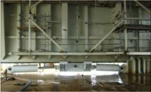
SKIDDING CYLINDER INSTALLATION
